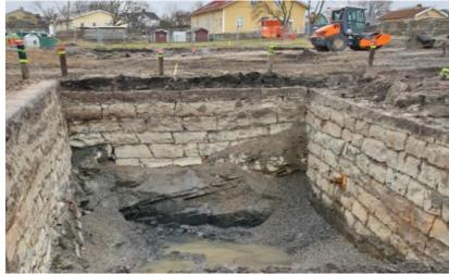
The goal of the clean-up was to remove the contamination in the source area and thereby avoid potential vapor intrusion and indoor air issues. An 8,600 ft<sup>2</sup> area to 164 ft below ground was defined as the source area to be remediated. The geology at the site consisted of 16 ft of overburden underlain by fractured granite with a maximum estimated total porosity of 0.5%. The water table was located approximately 6 ft bgs.
