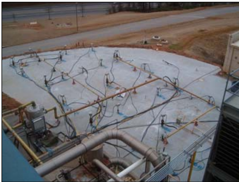
Figure 4. Completed ISTD system.
