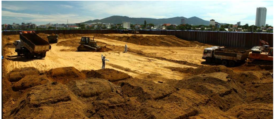
Placing contaminated soil and sediment in containment structure
