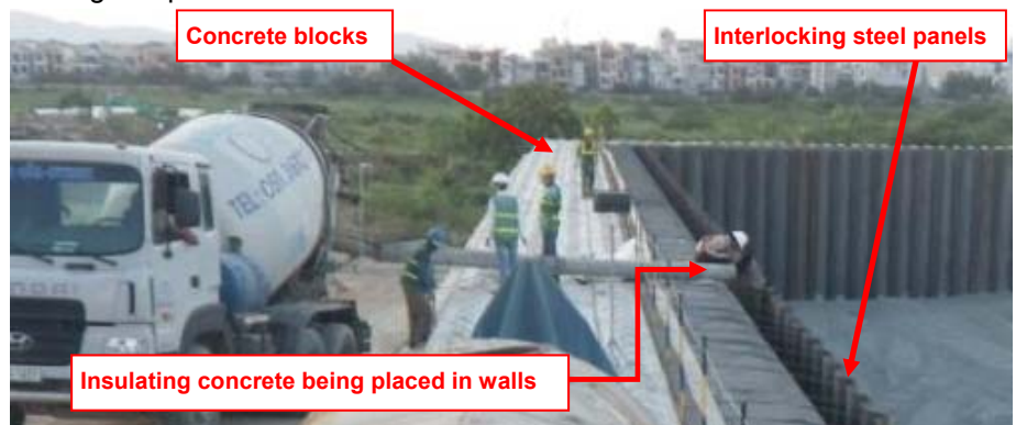
Pouring insulating concrete into the containment structure walls
