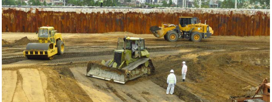
Loading and compacting contaminated soil into the treatment structure (Photos: TetraTech)
