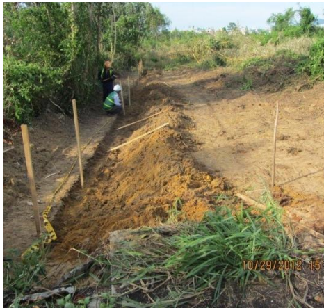
Installation of Silt Fencing (Photo: CDM Smith)
