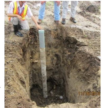
Test pits in pile structure (Photo: CDM Smith)
