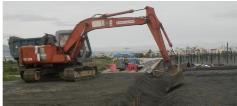
Placing gravel on top of the pile structure
